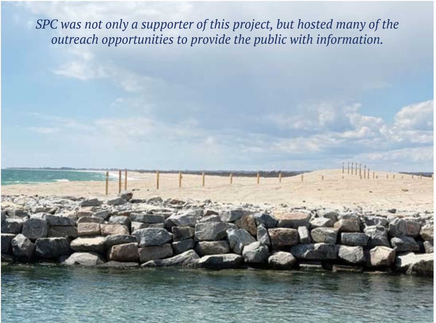
ABOVE, SHORED UP DUNES WILL REINFORCE THE INTEGRITY OF THE WESTERN WALL OF THE BREACHWAY.
