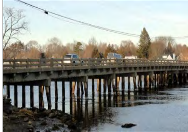
Central Bridge 182 in Barrington will be rebuilt with features to increase its resilience to sea level rise. (Photo Credit: RI DOT)
