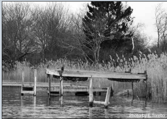
The high storm surge from Hurricane Sandy, on top of a full-moon spring tide, caused significant damage to private and commercial docks within Ninigret Pond. Center photo: Green Hill Pond. Right photo: Jim's Dock, Pt. Judith Pond.
