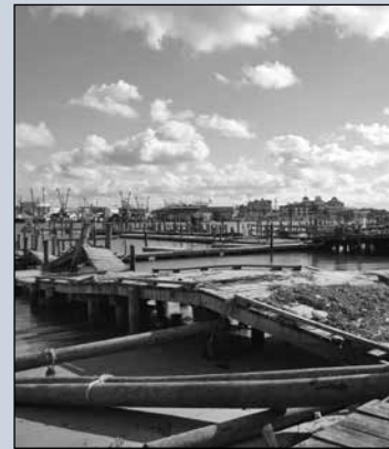
The high storm surge from Hurricane Sandy, on top of a full-moon spring tide, caused significant damage to private and commercial docks within Ninigret Pond. Center photo: Green Hill Pond. Right photo: Jim's Dock, Pt. Judith Pond.
