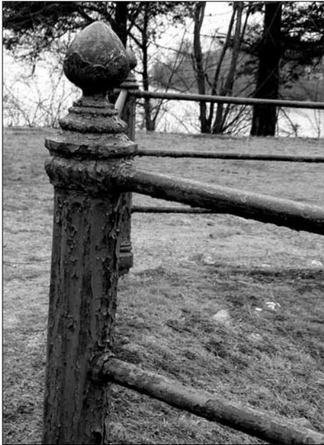
A section of the historic iron fence with badly peeling lead paint. The fence surrounds the old site and is over 800 feet long
